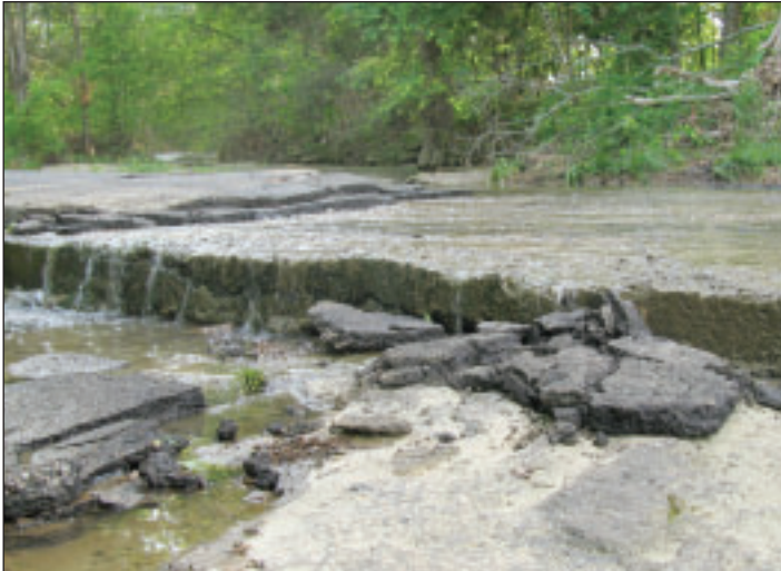
PHOTO BY DARYL K. TABOR Twenty county roads were damaged from flash flooding in the early morning hours Friday. Several layers of pavement along a portion of Cave Springs Road, above, were washed away down to a concrete slab along a creek bed.
